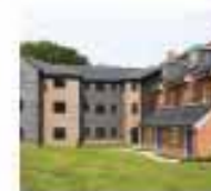
Faniers Walk Mildenhall Station
